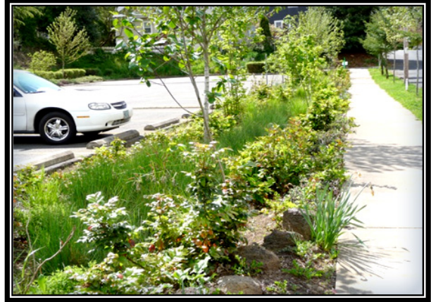
Parking Lot Sidewalks with Stormwater Bioretention Area
